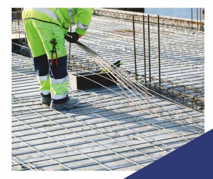
NJR Steel's reinforcing mesh is manufactured from hard-drawn wire and deformed cold-rolled wire with a minimum ultimate tensile strength of 510 MPa. It features a unique deformed wire pattern, known as the curry pattern, which facilitates superior bonding, stress-distribution and crack-width control.
